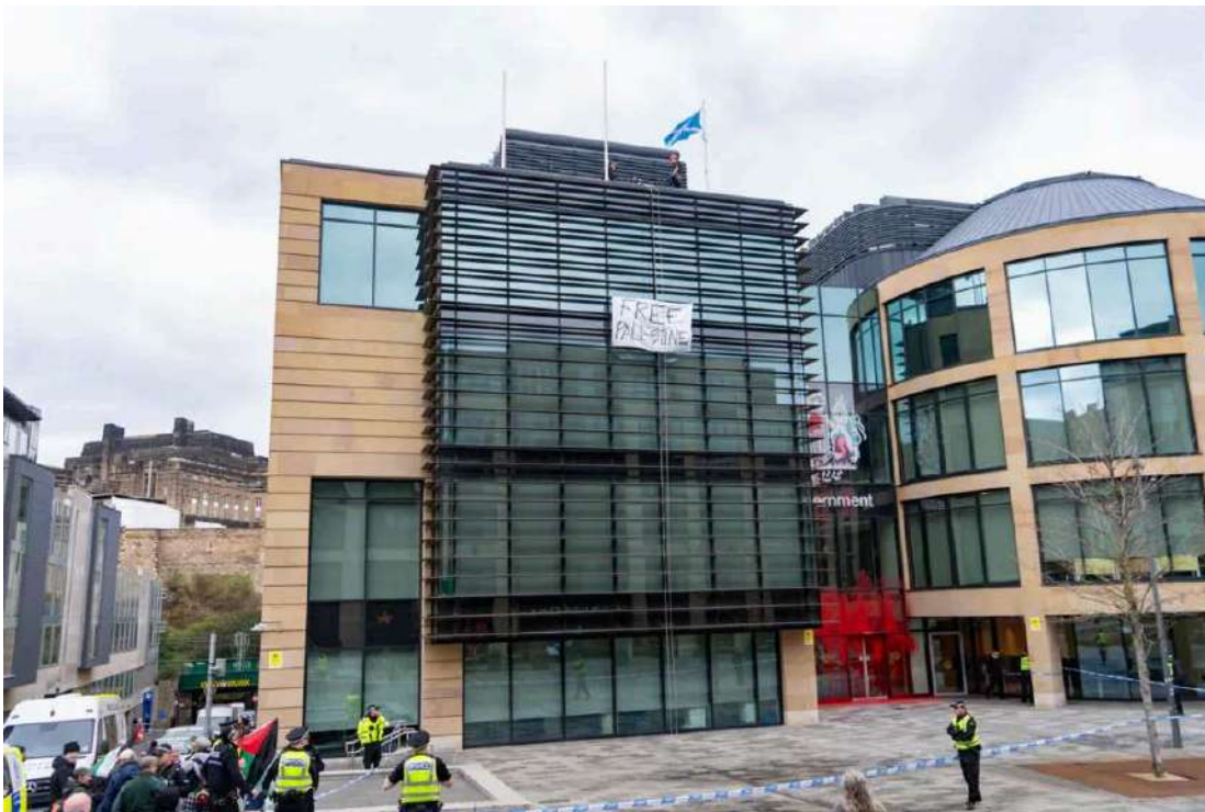
This is Rigged protesters scaled the UK Government building on Sibbald Walk in Edinburgh and daubed it with red paint.
